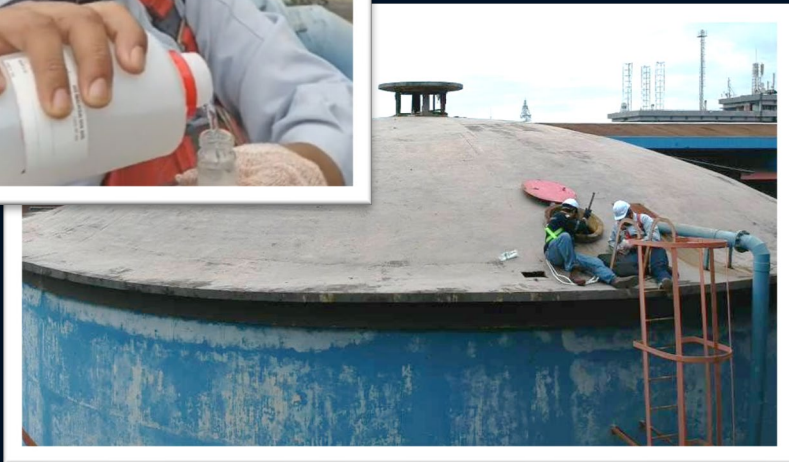
Satu Teknik's Inspection Team collecting water samples from a water tank
